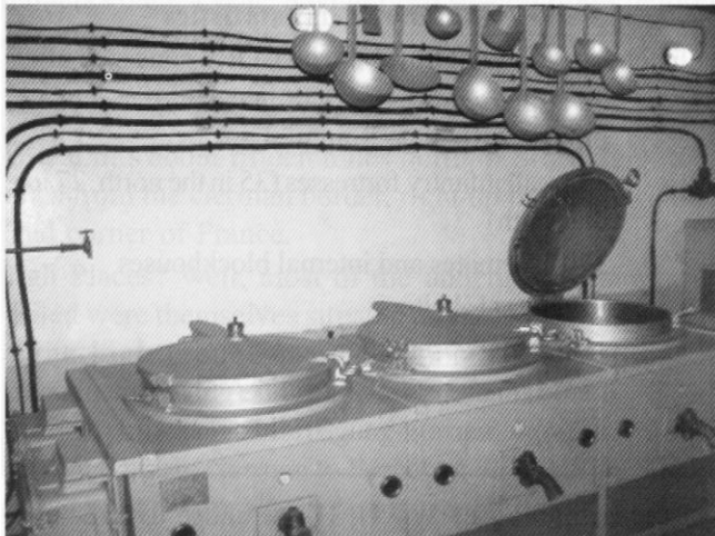
The main kitchen at Maginot Line 'Gros Ouvrage' Fort Schoenenbourg
